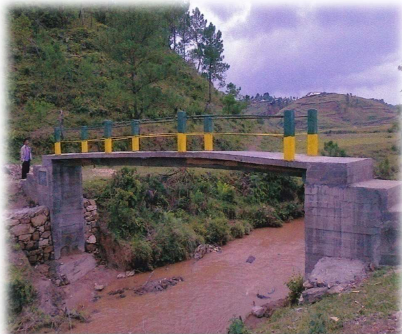
5. FOOTBRIDGE, IWMP PROJECT VII, ENTRY POINT ACTIVITIES
