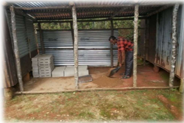
Hollow Block Making at Nongliput
